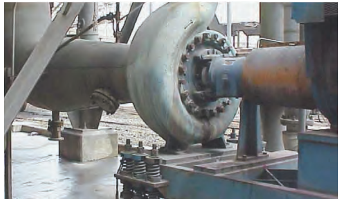
Installation for a difficult high-temperature service. Spring-mounted baseplate provided to compensate for thermal expansion.
